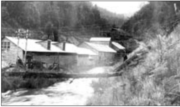
**Figure 10:** The Mount Bischoff Company's centrifugal dredge operating in the North Bischoff Valley, 1928. A high-pressure hose washed alluvium into a sump. Suction pumps on the dredge deposited tin ore in sluice-boxes. (Photo by RE Smith photo courtesy of Charles Smith)
